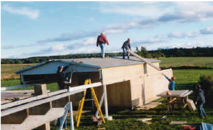
Over the following summer months, making full use of the skills of members of Toronto Centre, the exterior walls of the observatory were constructed, using 2 x 4 studs and 19mm (¾") and 13mm (½") plywood cladding. The walls were bolted to the structural steel frame. Closely spaced electrical receptacles were installed in the walls of the observatory and provisions were made for data ports.
